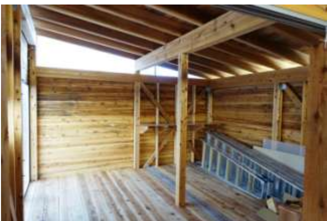
(63)水屋南側内壁
